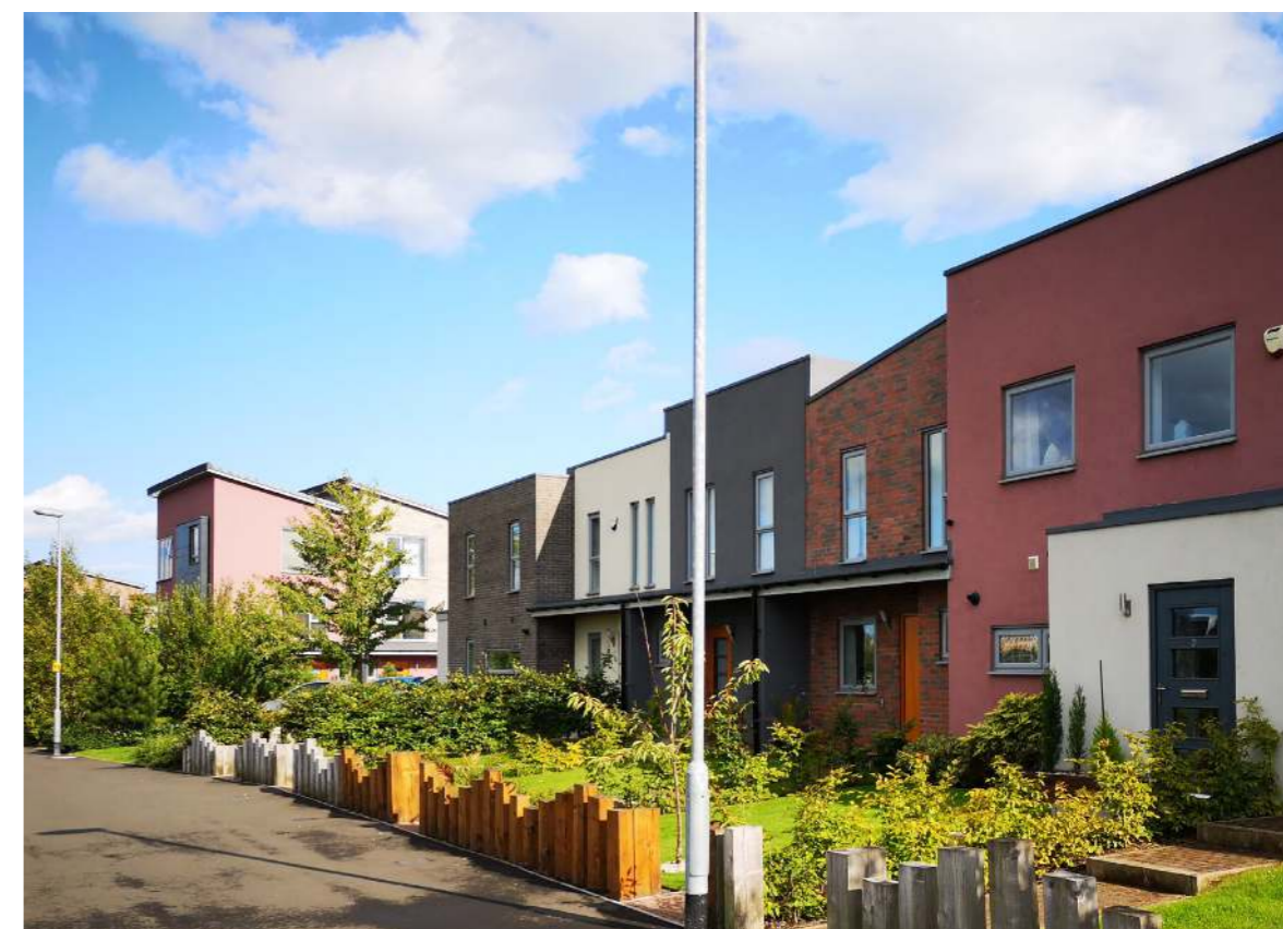
Fig 24: Staithe housing, Gateshead. Front gardens with low fences and varied planting creates a buffer between houses and street, whilst clear visibility of entrances and front windows help animate the street.
