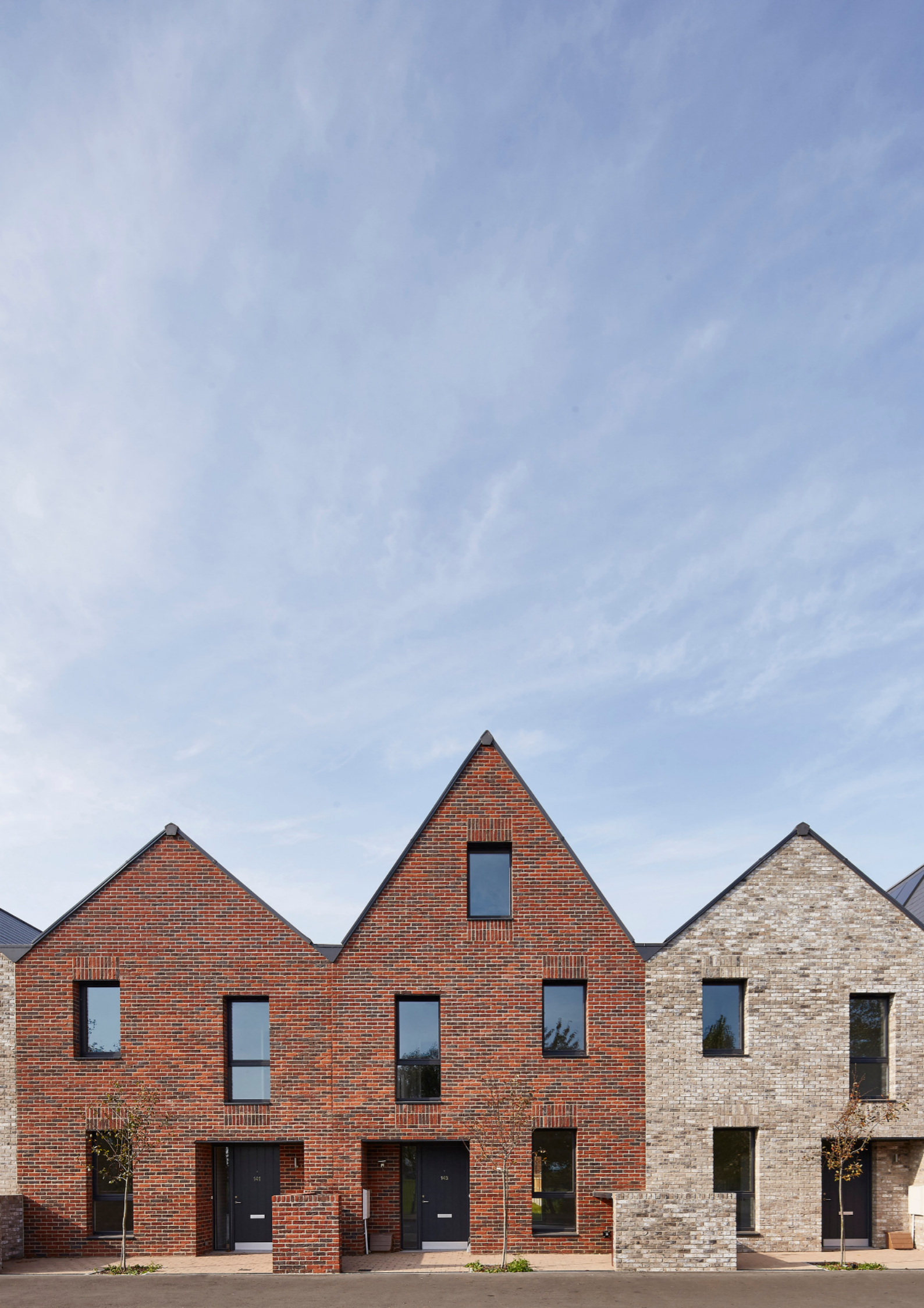
Fig 46: St Chads, Thurrock Council, Essex by Bell Philips Architects. A tight budget limited the team to UPVC windows. The detail used fixes the frame behind the brick reveal to reduce the typical bulky mass of UPVC windows. The windows are also colour matched to avoid the typical glossiness of white UPVC.
