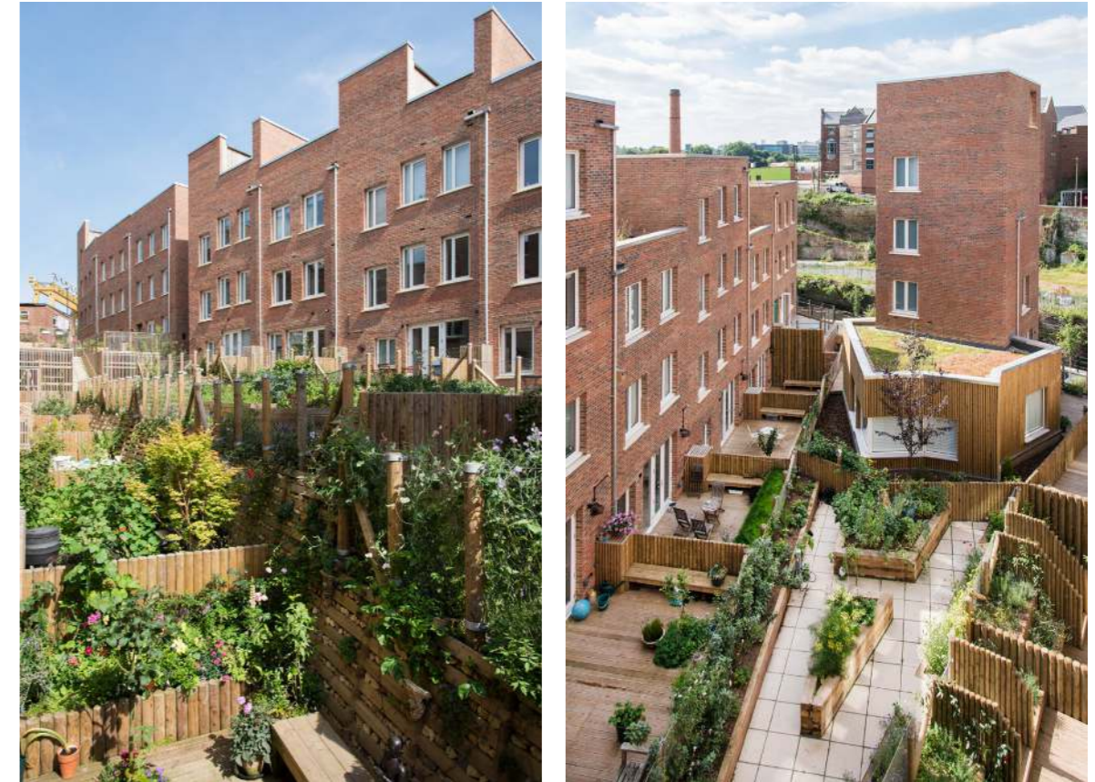
Fig 17: The Malings, Newcastle Upon Tyne - by Ask Sakula Architects and developed by Igloo. Townscape is created through a continuity of materials that reflects the local industrial context without slavishly imitating the form or scale.
