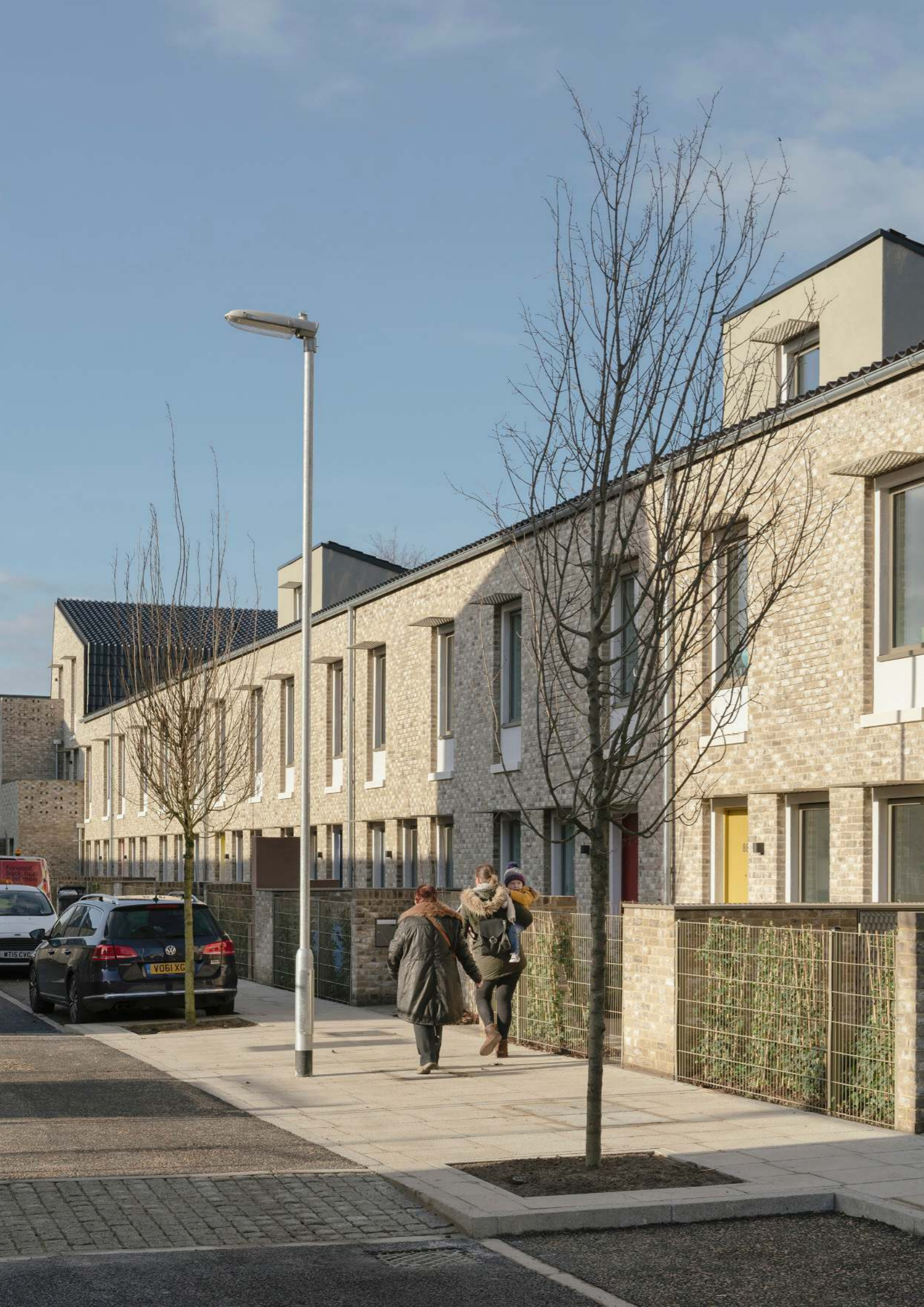
Fig 54: Goldsmith Street, Norwich by Mikhail Riches Architects for Norwich City Council. The development achieves Passivhaus house standards using fabric first principles including solar shading to reduce heat gain to some windows. Awarded the RIBA Stirling Prize 2019.
